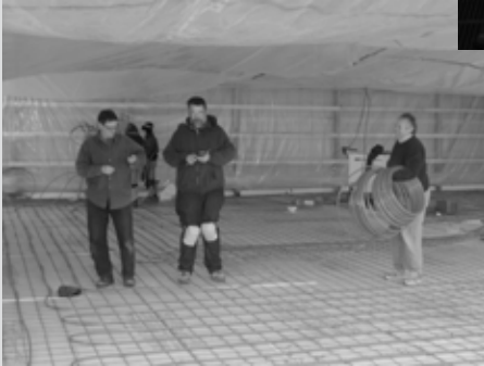
Crew installing floor heat
